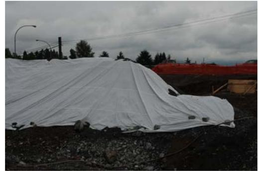
**10. Dewater to a contained part of the site and allow it to infiltrate into the soil:**
