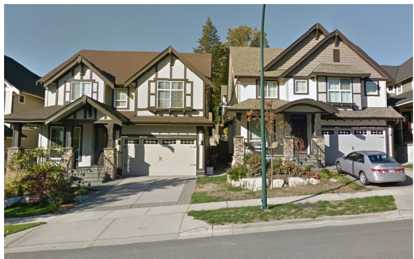
Exposed basements screened with landscaping (b).
