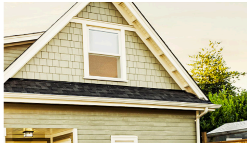
High quality siding, trim, and detailing (a)
