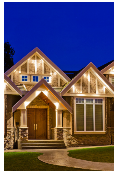
Avoid this - angled upper soffit lighting
