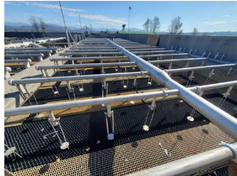
Trickling Filter media replacement
