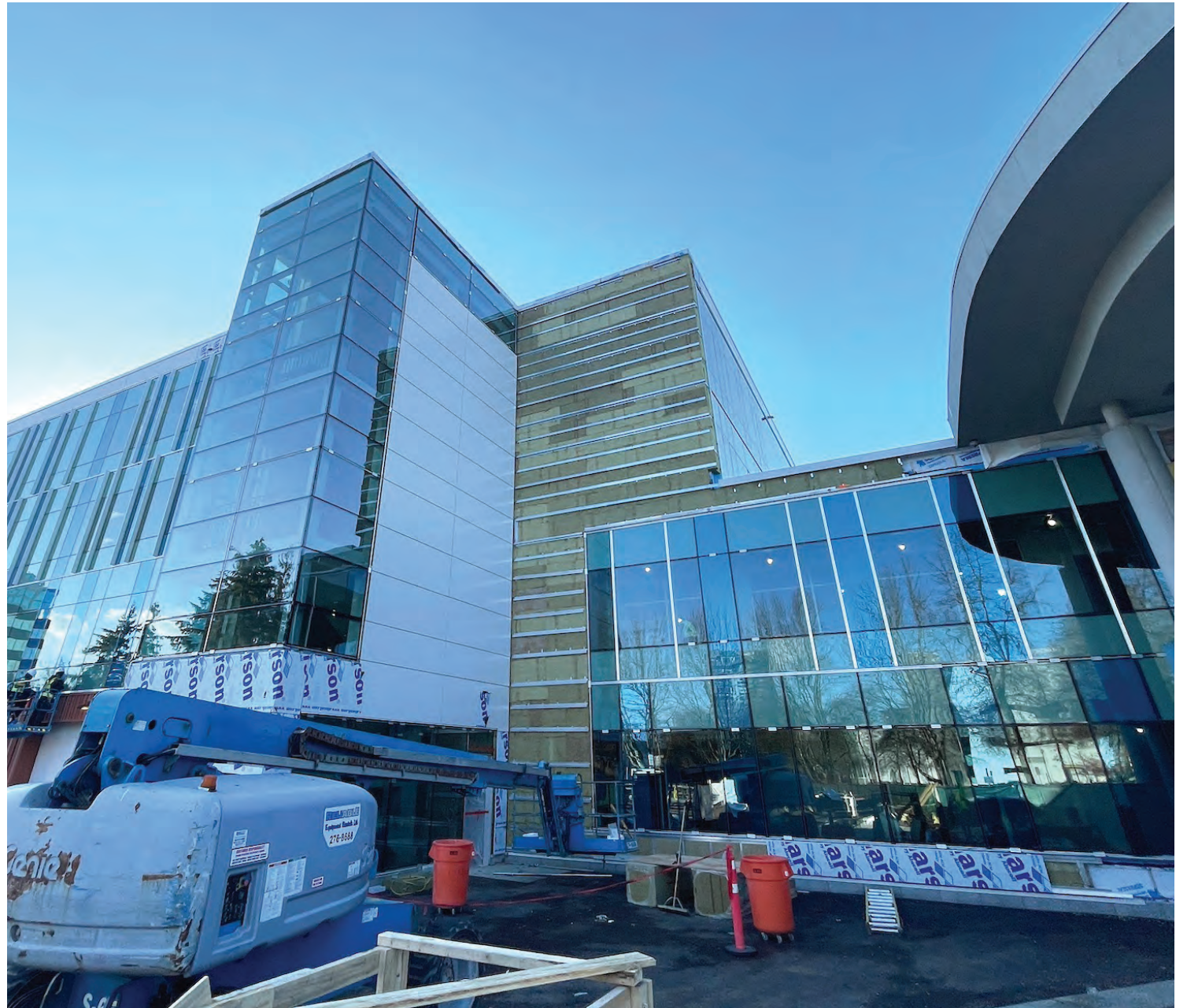
A 105,000-square-foot addition to the Abbotsford Police Department is nearing completion and is expected to be ready for occupancy in March 2025. (Abbotsford Police Department)
