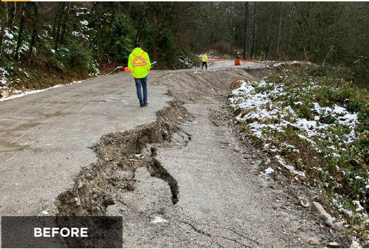
ROAD REPAIR: NORRISH CREEK FOREST SERVICE ROAD
