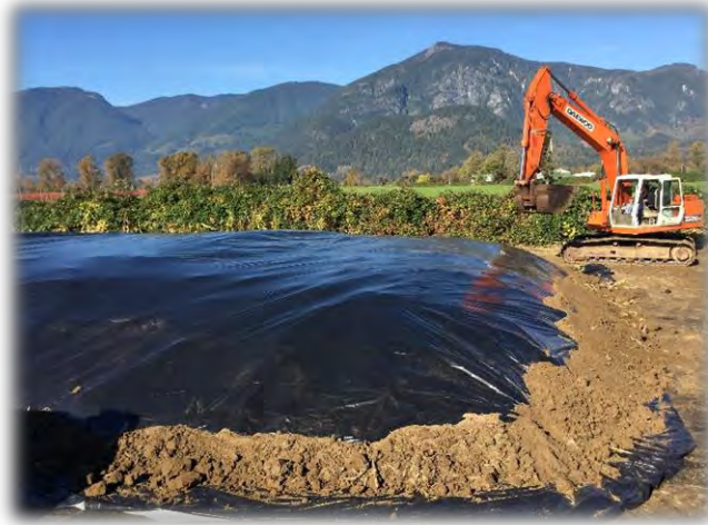
Photo 1 Class A biosolids stockpile at 1233 Kilby Rd.
