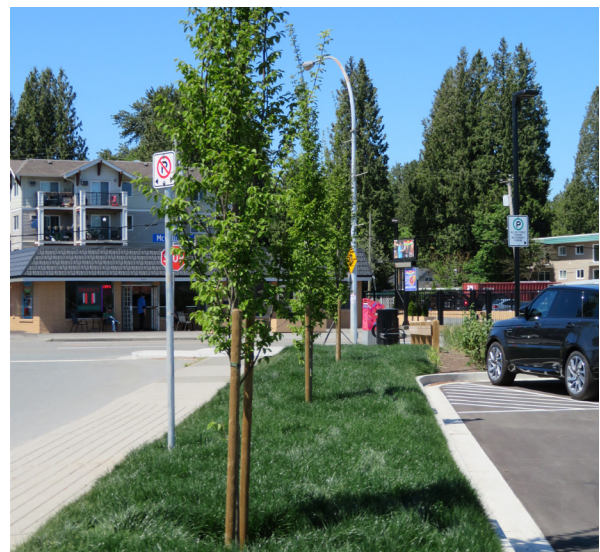
An enhanced streetscape and surface parking area with stormwater management was installed as part of the Jubilee Park Improvement Project.
