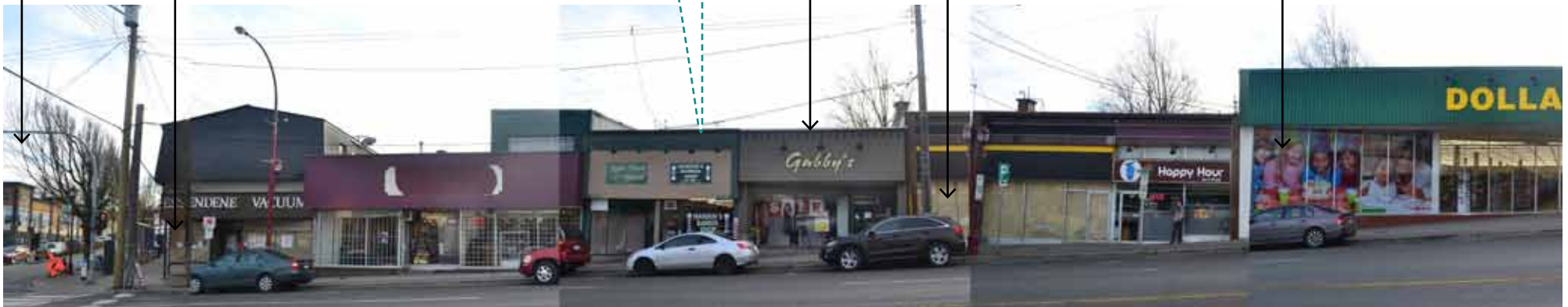
Figure 56. Photo Montage: Essendene Avenue South Side
