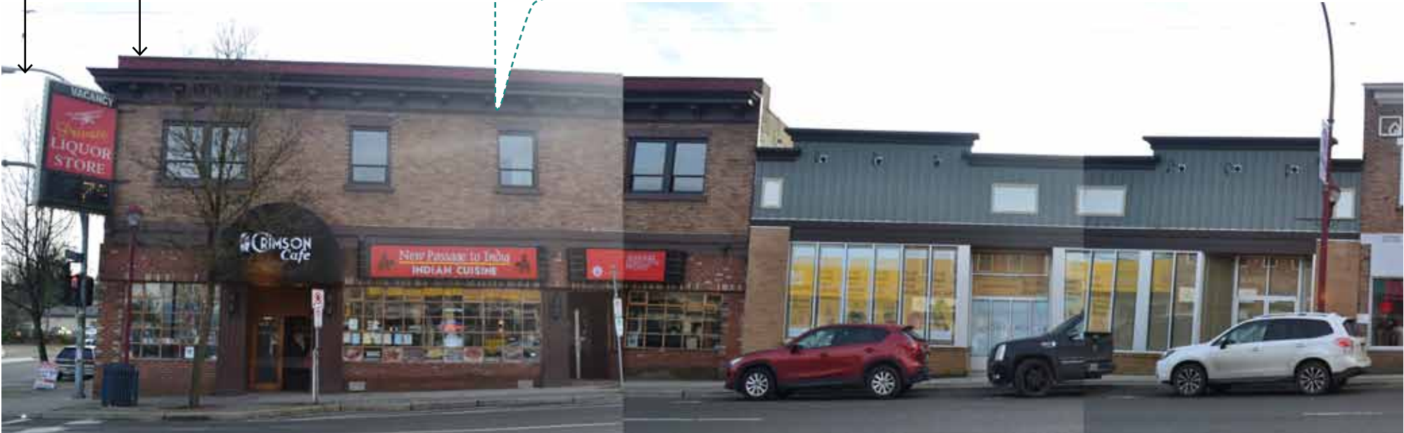
Figure 55. Photo Montage: Essendene Avenue South Side
