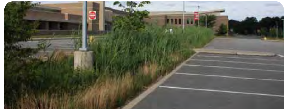
Situating raingardens adjacent to surface parking is a simple way to reduce the impact of large paved surfaces. Image: Montgomery County Planning Commission.
