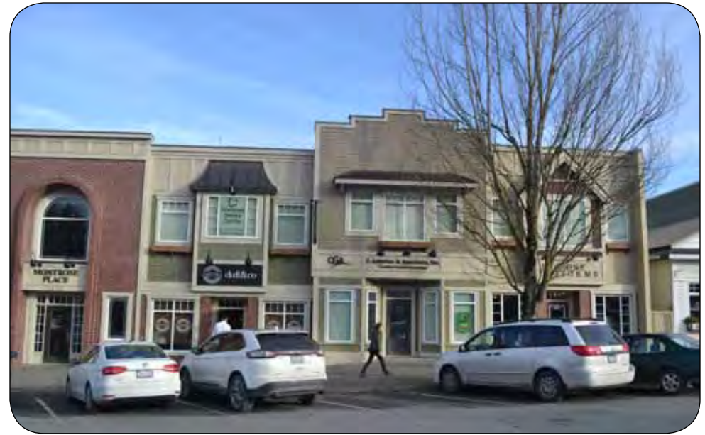
Figure 31. Montrose Avenue development (2009)
