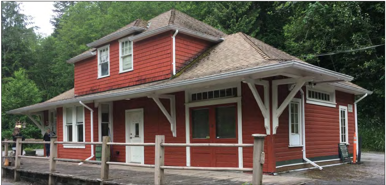
Figure 6 – C.P. Rail Station
