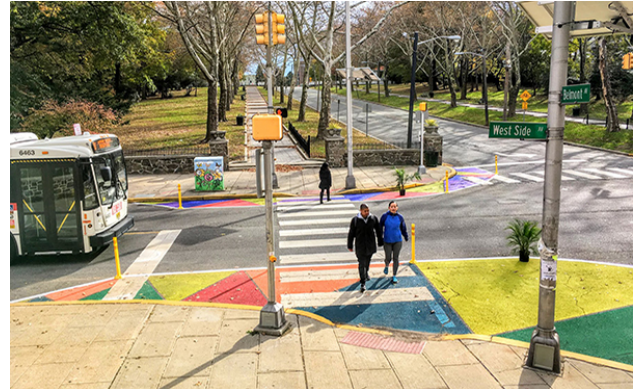
Figure 15 - Temporary Curb Bulge (photo credit: Street Plans Collaborative)
