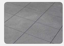
Indicative saw cut design in boulevards (Refer to plans for actual saw cut design and dimensions)
