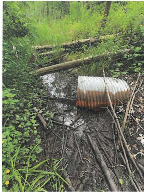
Photograph 2 – Illustration of unmapped CMP culvert crossing of Hwy 11 under low water conditions (June 2021).
