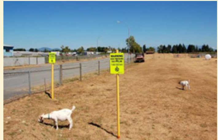
Gas Pipeline at Queen St & Marshall Rd
