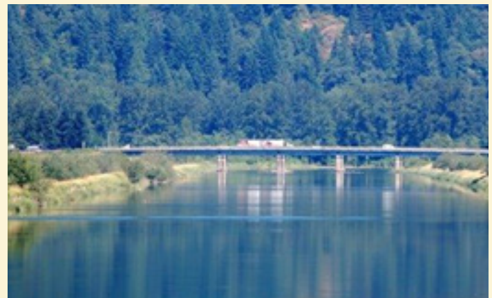
TransCanada Highway over Vedder Canal
