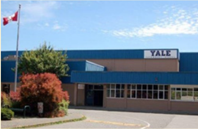
Flat Roof at Yale Secondary School
