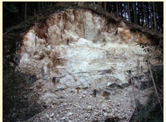
Slide Damages Abbotsford Water System (Source: Abbotsford News)
