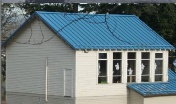
South Poplar Elementary
