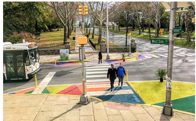
Figure 11 - Temporary Curb Bulge
