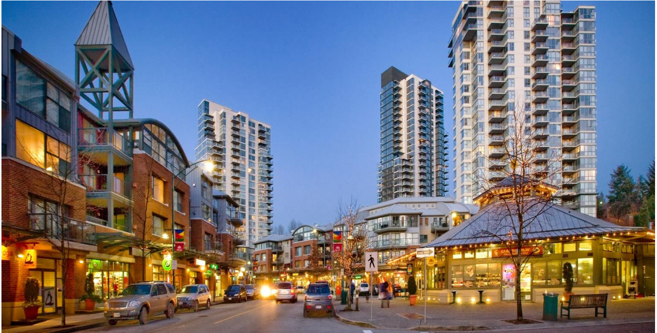
Figure 9 - Commercial Street in Newport Village, Port Moody
