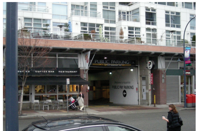
Figure 18: Access to underground parking should be architecturally integrated to minimize the visual impact.
