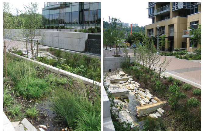
Figure 30: Weirs and check-dams help to slow the flow of water and facilitate infiltration
