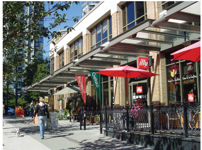
Figure 21: In Abbotsford’s climate, transparent material provides protection from the rain while still allowing sunlight to reach the sidewalk.
