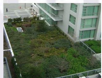
Victoria Marriot Inn's green roof
