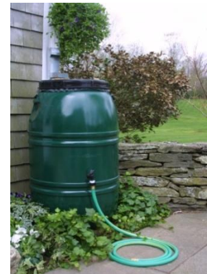
Rain barrels for rainwater harvesting
