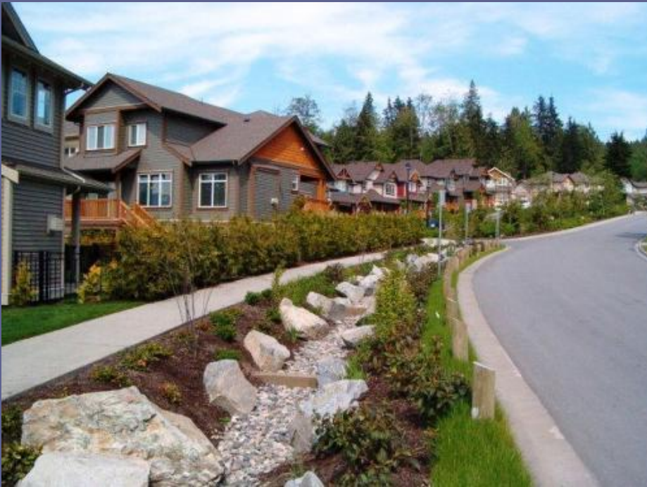
Rain gardens used in Silver Ridge provide a stormwater management function while separating foot and vehicle traffic and creating a visually appealing streetscape.
