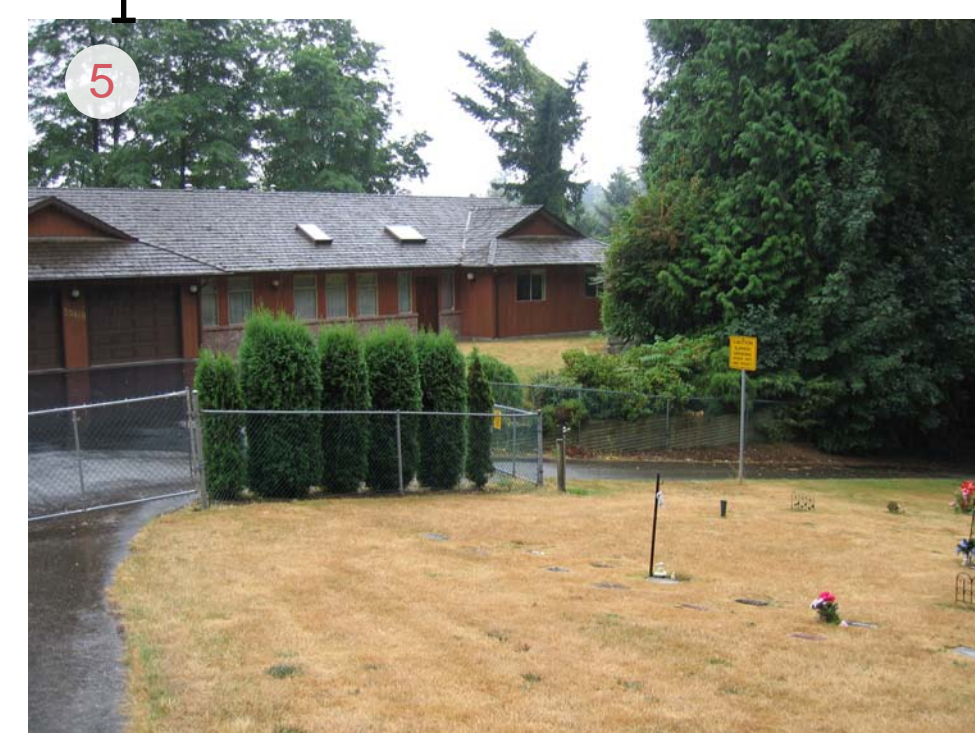
South Property Line - Service road is rarely used - Lack of separation between cemetery and residential area
