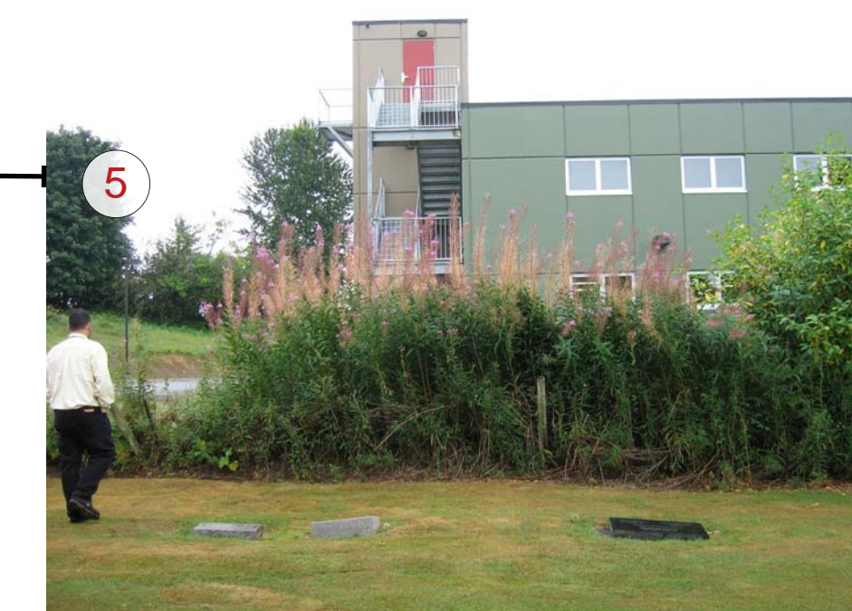
Neighbouring firehall to the east - Insufficient separation and screening
